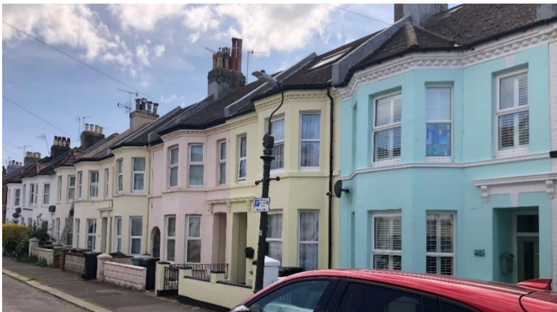
Figure 6: Photo of inappropriate PVCu casement windows
